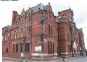
North East corner 2004
