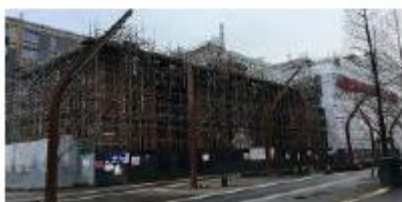
North East corner 2021
