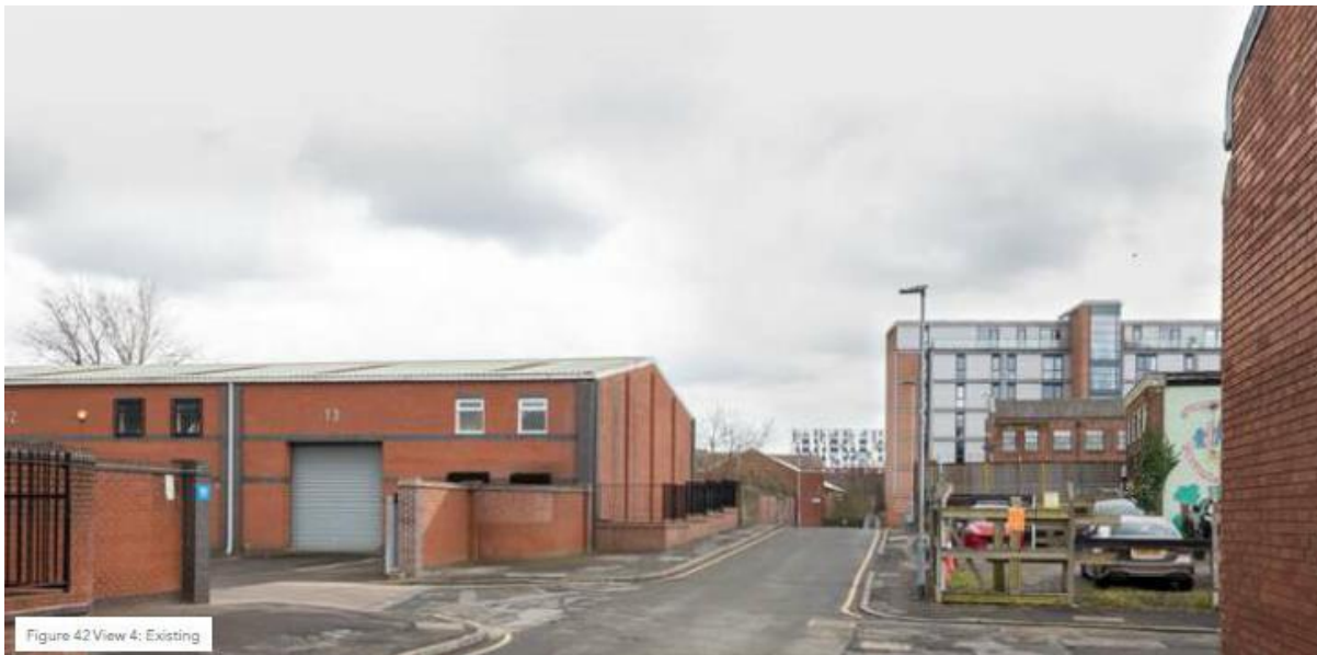
North south along Poland Street – existing
