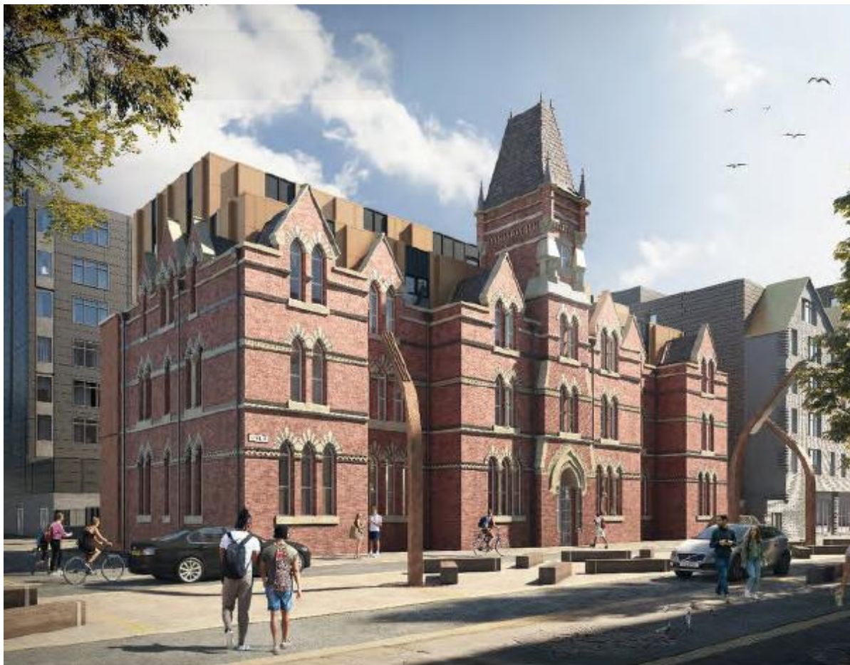
Image of the refurbished building including retained and repaired façade (including central tower) together with roof top and rear extension
